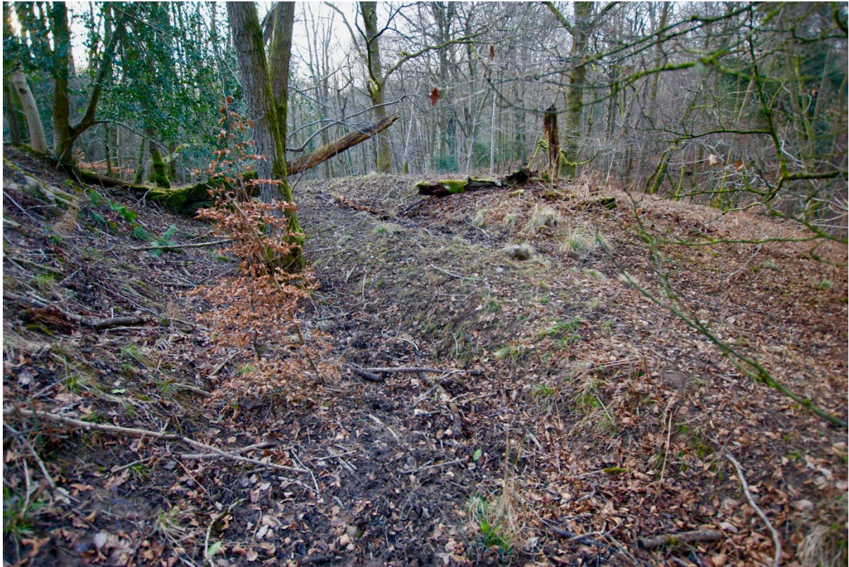
Figure 11. On the left is the large forestry bank in the centre is the bed of the tramroad ditched on either side
